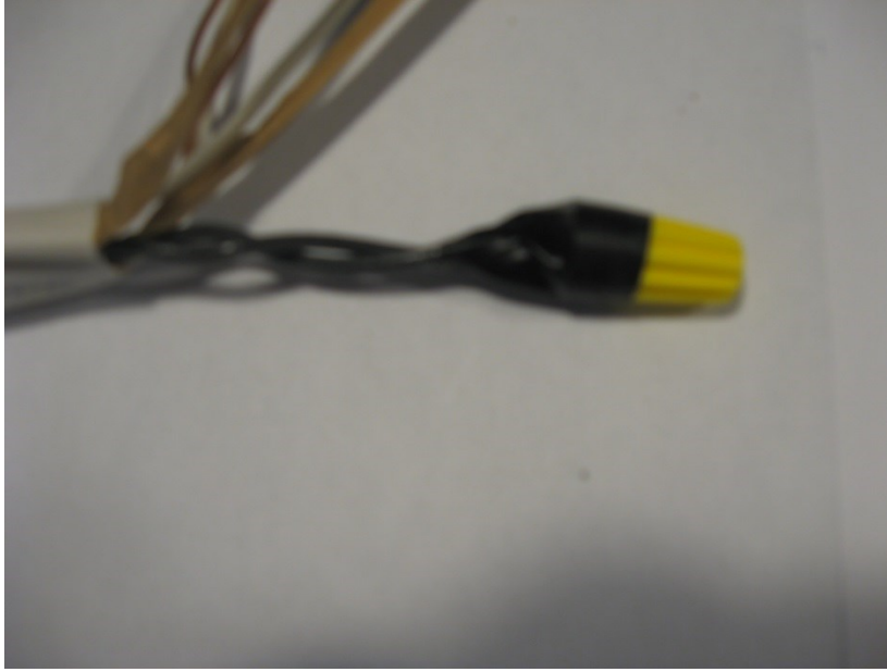
Figure 5. Apply electrical tape to cover the base of the wire nut and the insulated wires.
