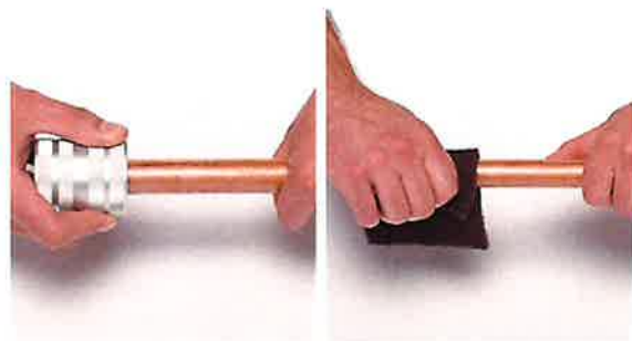
Following tube preparation steps 4 to 8 in the RLS installation instructions is important for preventing leaks.
