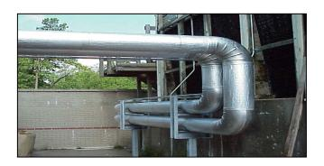
Alumaguard All-Weather is typically applied to faced fiberglass board, rigid isocyanurate foam board with facing, or unfaced extruded polystyrene foam board.
