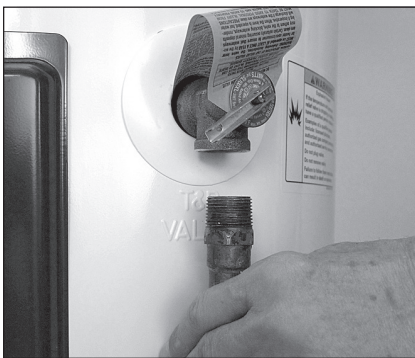
Removing the T&P Relief Valve discharge pipe.
