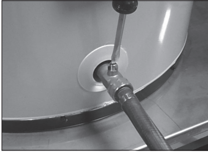
Draining the old water heater.
