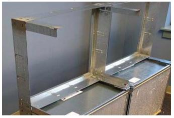
Figure 36: Insert HEPA Filter into Frame, until the Gasket Comes in Contact with the Holding Frame
