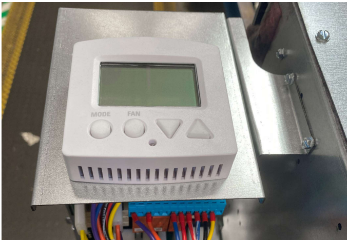
Figure 33. Thermostat unit-mount
