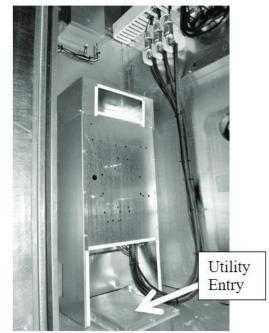
Figure 28 - Back View of Utility Entry and Power Switch from Control Compartment (55, 65 and 75-140 ton Units)
