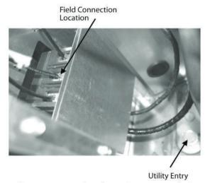
Figure 27 - Back View of Power Switch from Compressor and Control Compartment (6-50, 60, and 70 ton Units)
