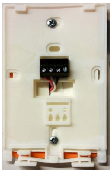
Figure 3 Completely cover all holes in the Microset 4 backplate to safeguard against air infiltration.
