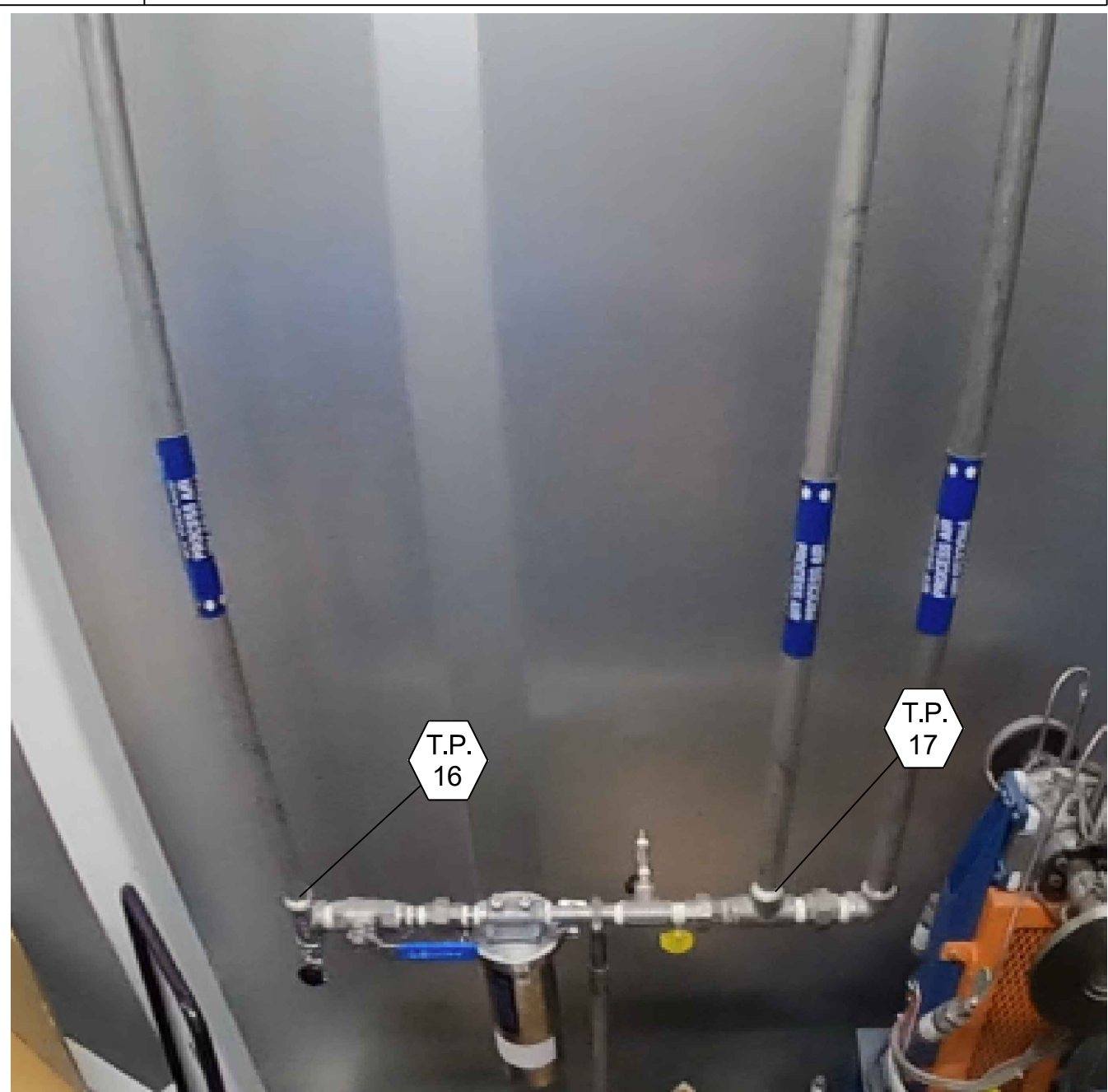
TIE-IN 16 - 17 - LOOKING NORTH
