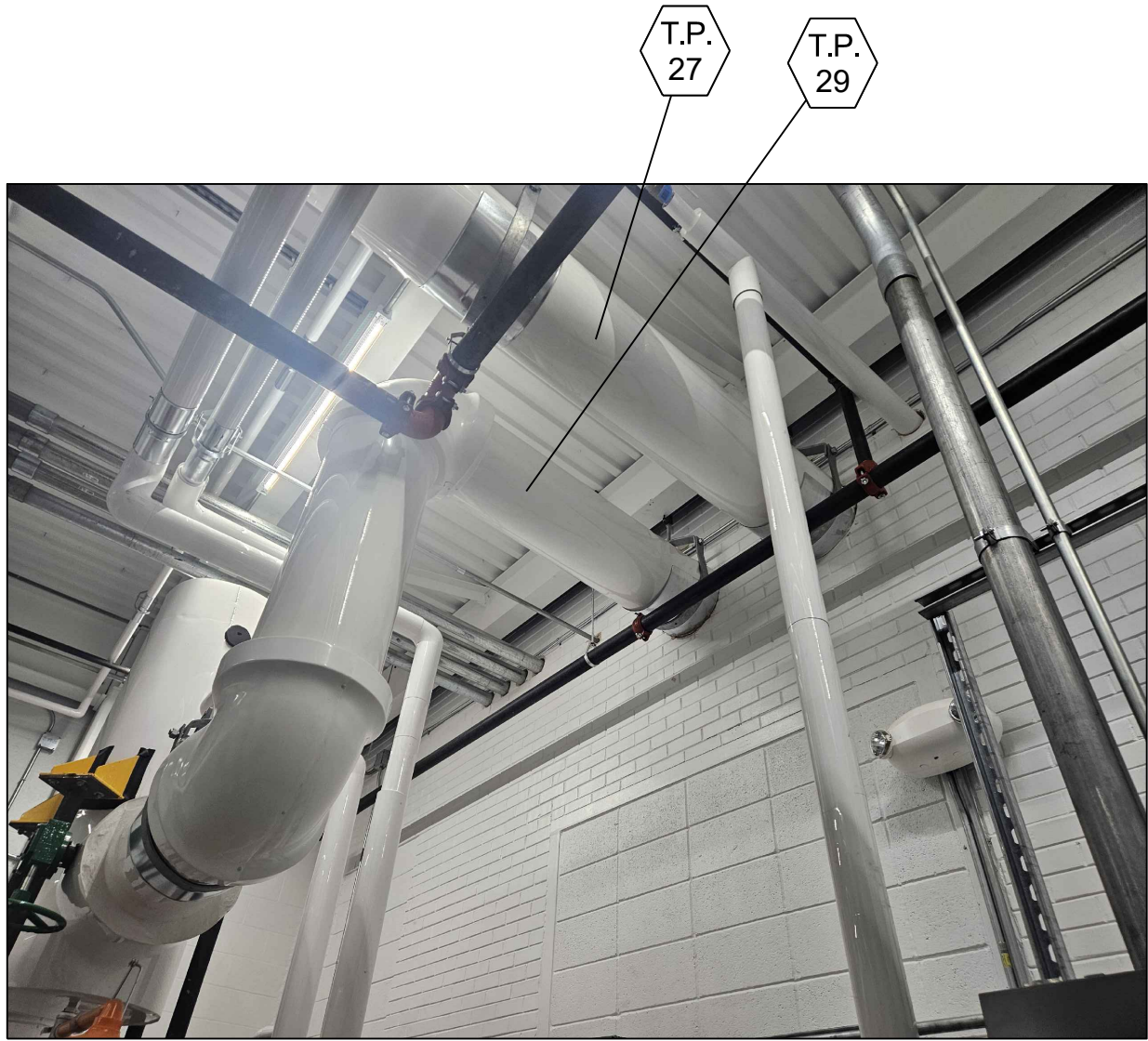
TIE-IN 27, 29 - LOOKING NORTH
