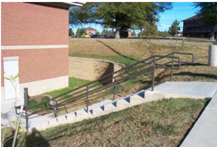
Concrete masonry retaining wall at Building 952
