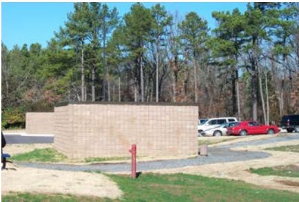
Effective screening enclosure
