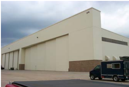
Aircraft hangars with masonry wainscot
