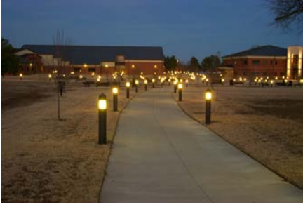
Bollard lighting should be placed in paving for ease of landscape maintenance
