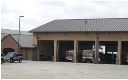
Example of well scaled fascia
