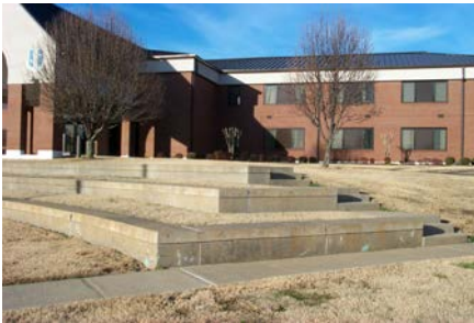
Retaining wall at Building 1250
