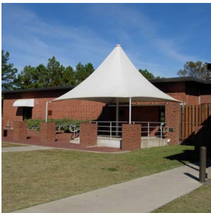
Tensile structure at Building 1080
