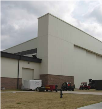
Masonry wainscot improves human scale of large building
