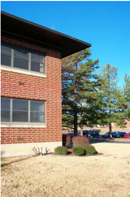
Overhang reduces solar heat gain
