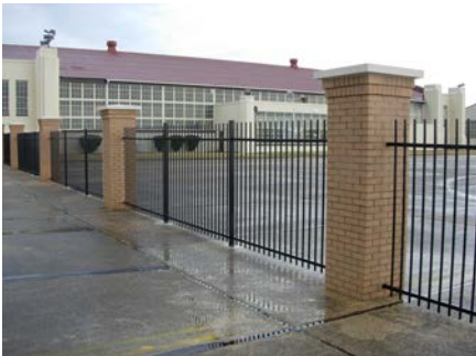
Security fencing at Maxwell AFB
