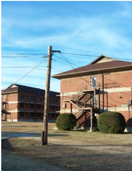
Power lines contribute to visual clutter
