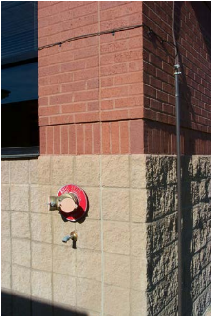
Brick above split-face CMU
