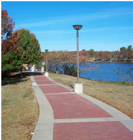
Brick pavers in concrete walkway
