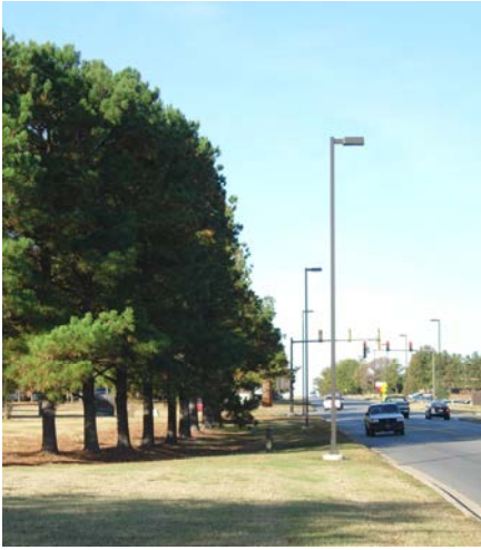
Effective roadway lighting
