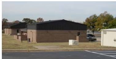
Buildings with gabled ends
