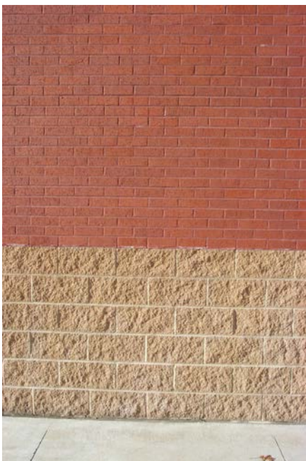
Brick and split-face CMU
