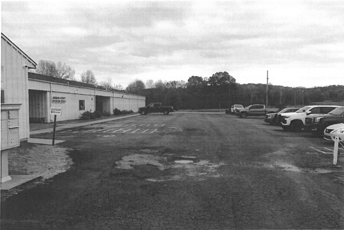
Parking Lot Between Building and Road
