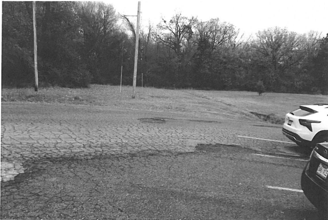
Rear Area Behind Existing Building
