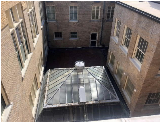
Photo #3 Lower central courtyard roof
