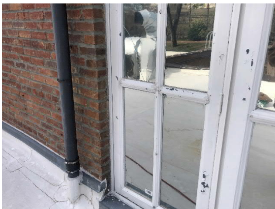
Photo #11 Metal drain pipe and windows.
