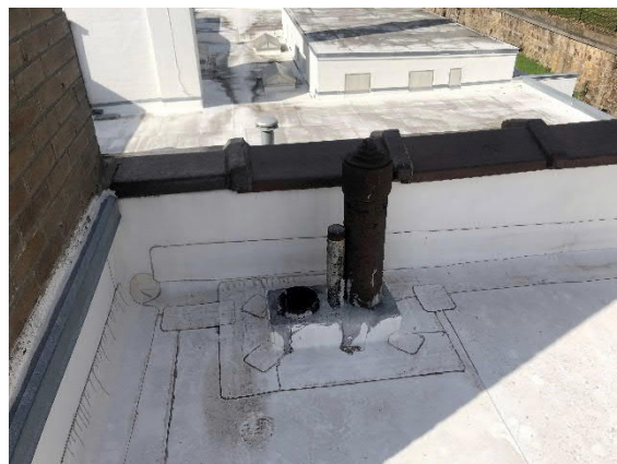
Photo #12 Roof penetration with remnant roofing tar.
