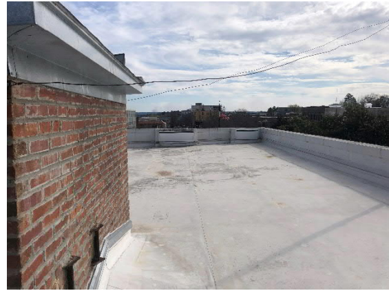
Photo #2 Overview of the roof.
