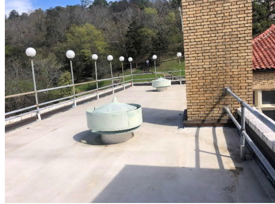
Photo #2 Overview of the roof.
