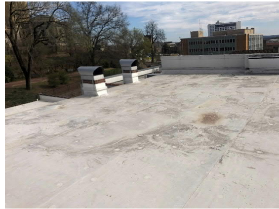
Photo #4 Overview of the roof.
