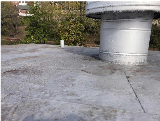
Photo #5 Roof vent.
