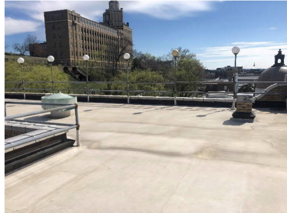
Photo #10 Overview of the upper roof.
