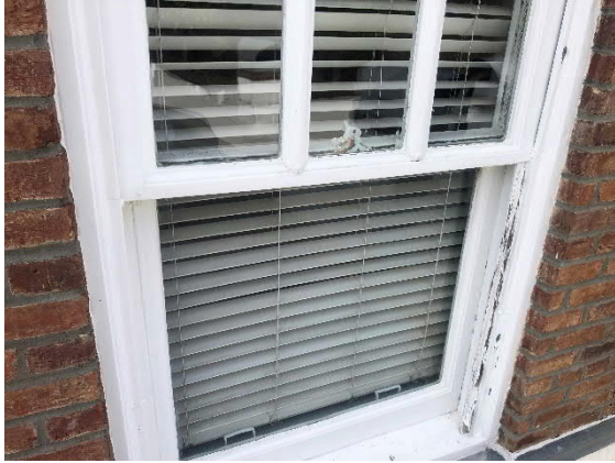
Photo #7 Example of window observed on roof.
