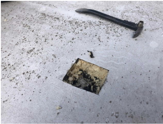
Photo #3 Example of roof core sample location
