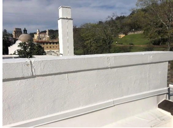
Photo #8 Roof parapet
