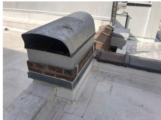
Photo #6 Roof vent.
