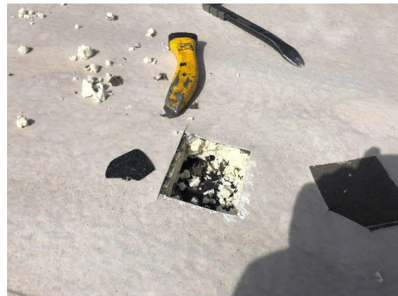
Photo #6 Example of roof core sample location.
