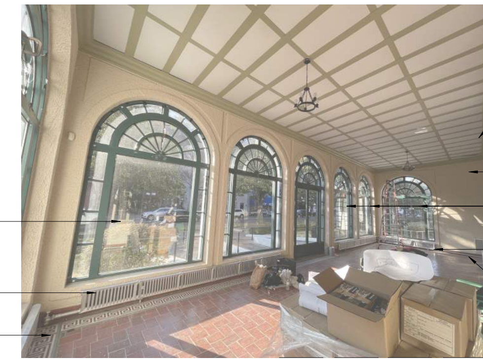
SUN PORCH 109, LOOKING WEST
