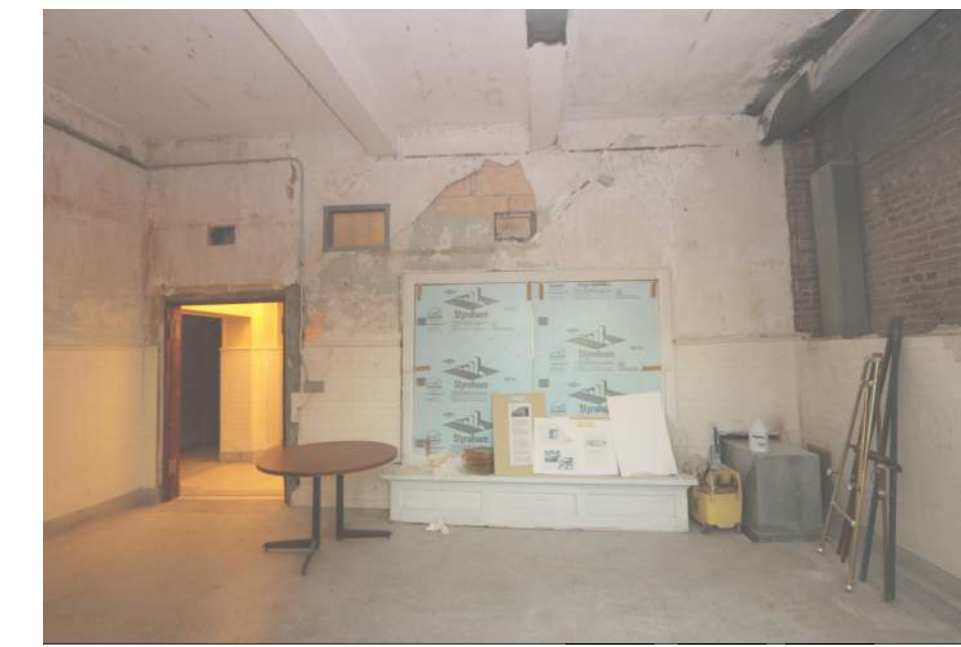
WOMEN'S COOLING ROOM 105, LOOKING WEST
