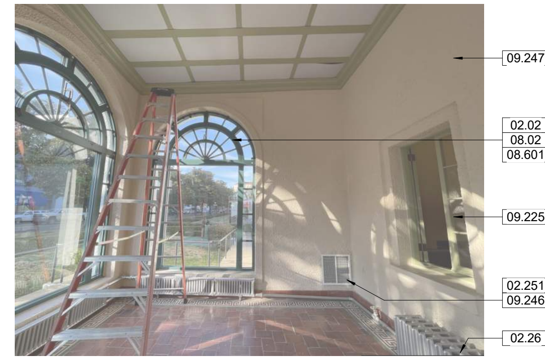
SUN PORCH 109, LOOKING NORTH
