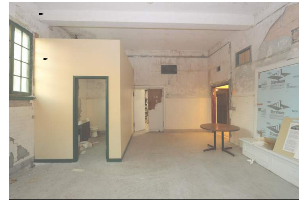
WOMEN'S COOLING ROOM 105, LOOKING SOUTH
