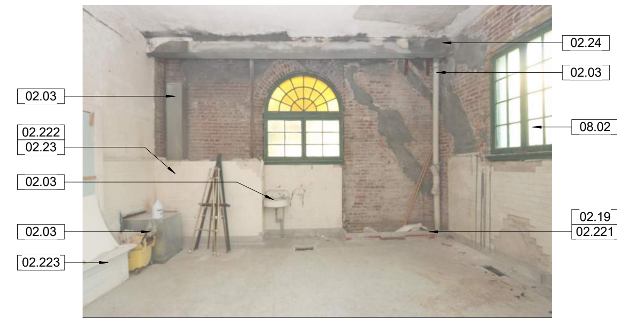
WOMEN'S COOLING ROOM 105, LOOKING WEST
