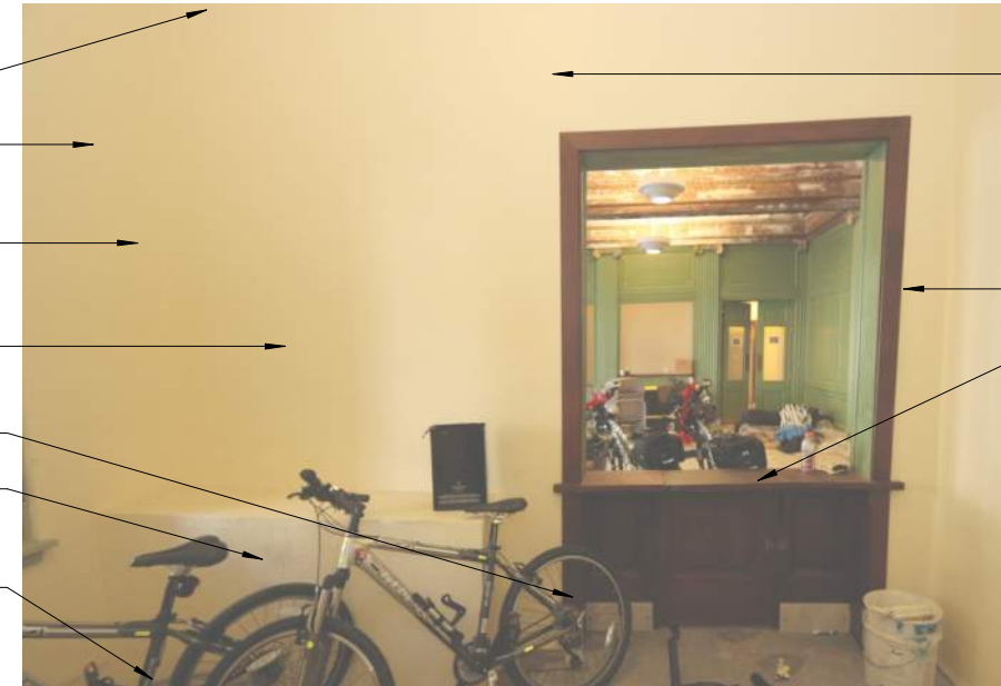
CLOAKROOM 117, LOOKING NORTH
