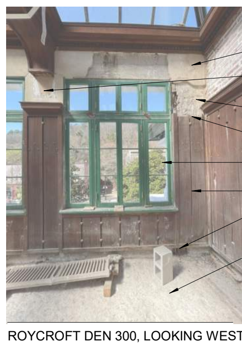
ROYCROFT DEN 300, LOOKING WEST
