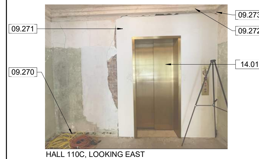
HALL 110C, LOOKING EAST
