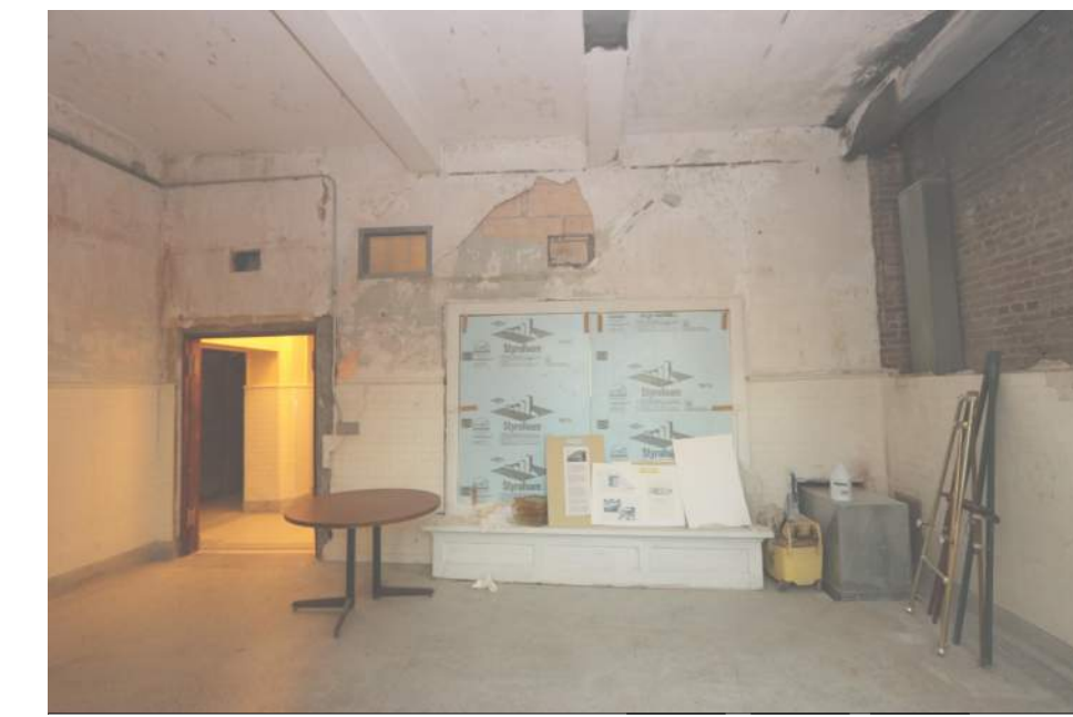
WOMEN'S COOLING ROOM 105, LOOKING WEST
