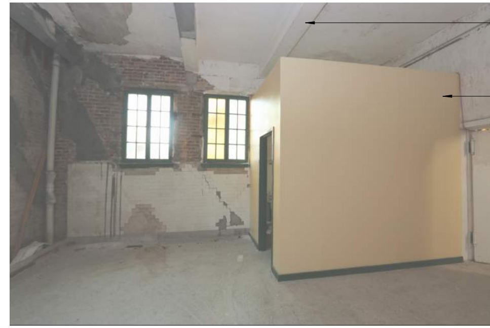
WOMEN'S COOLING ROOM 105, LOOKING NORTH
