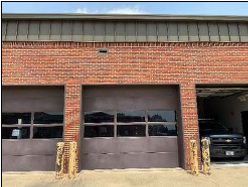
6 - B201 Infill South Doors
