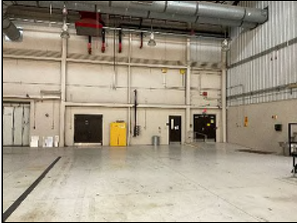
43 - B202 Hangar Bay 3 North Wall East Side
