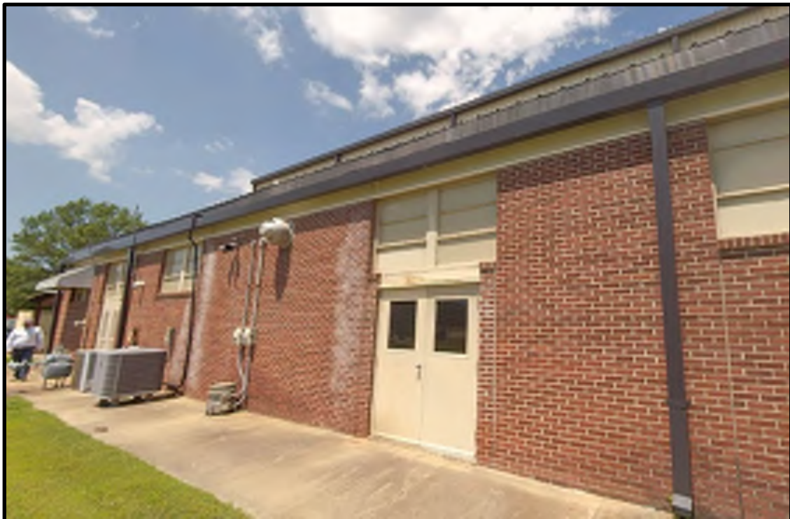
56 - B214 Exterior View #2
