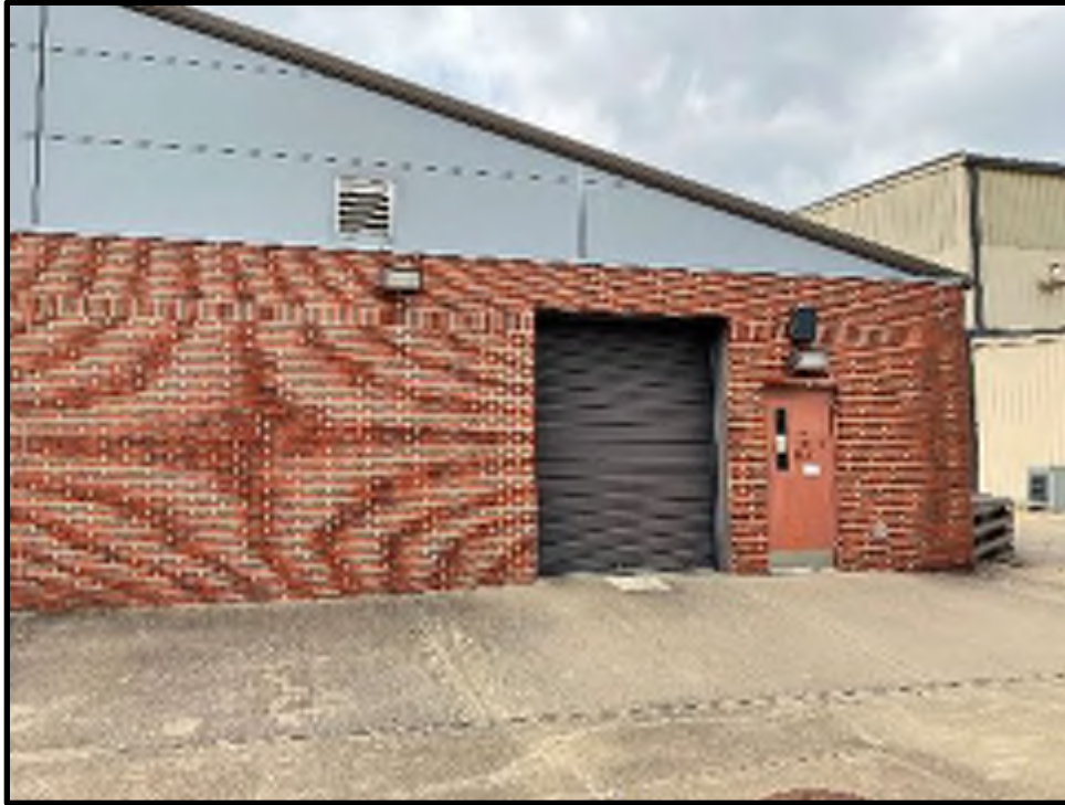
23 - B202 Exterior Tank Bay Doors
