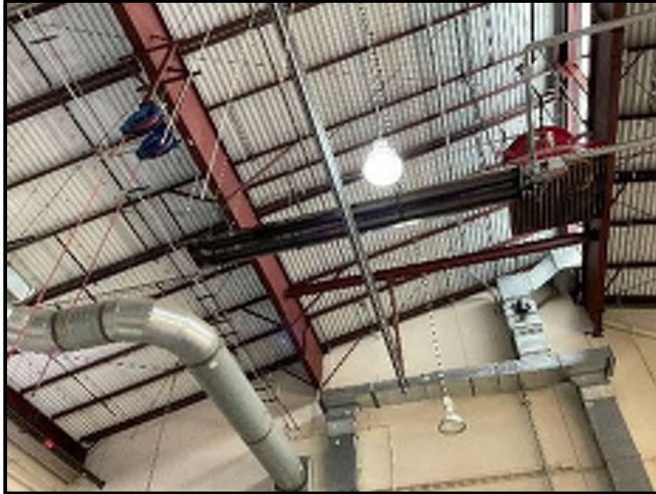
41 - B202 Hangar Bay 2 Ceiling
