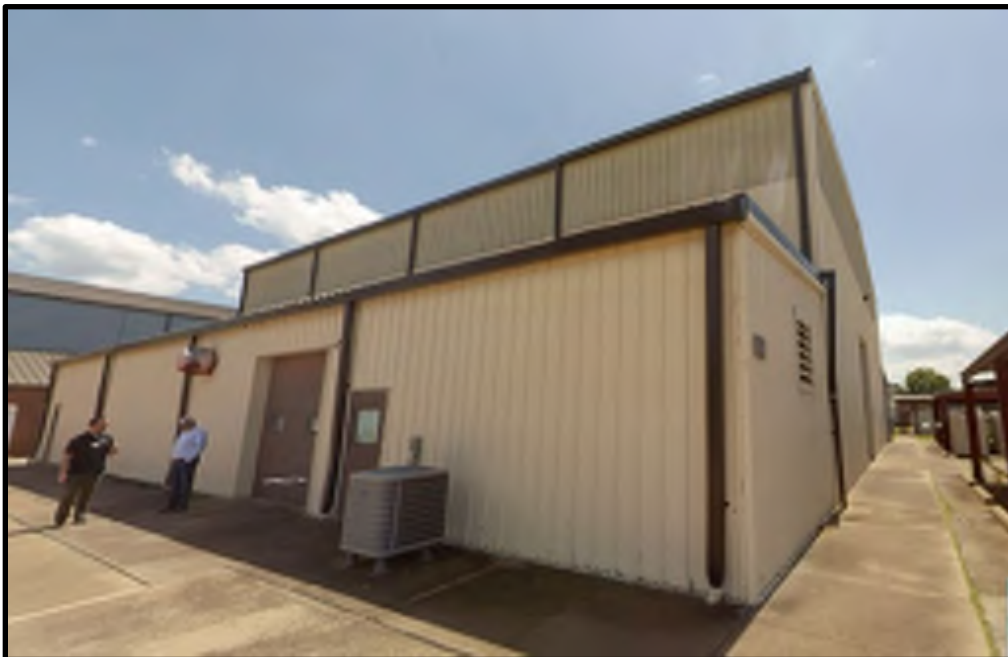
58 - B214 Exterior View #4
