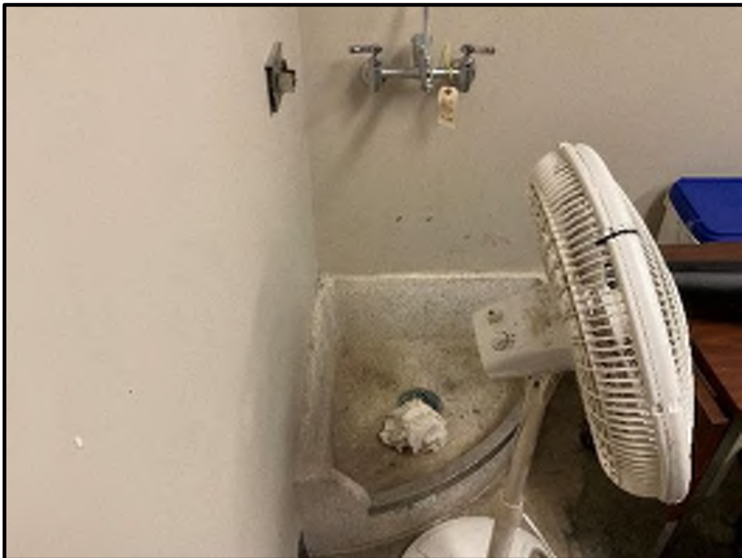
34 - B202 Existing Service Sink
