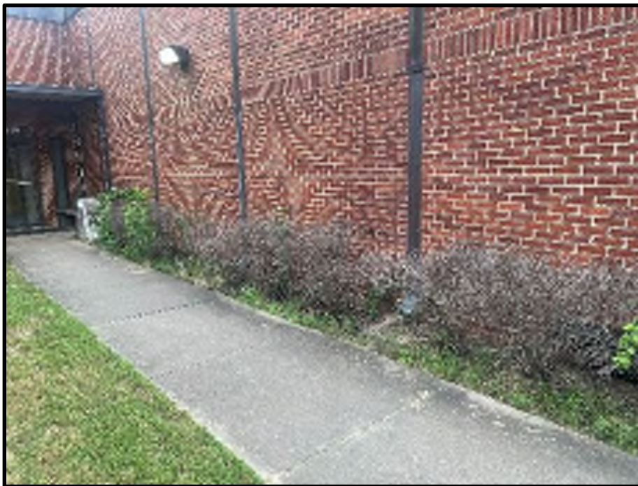
78 - B216 Downspouts by Addition
