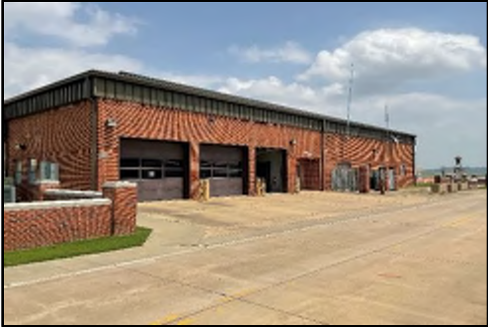
3 - B201 South Facade
