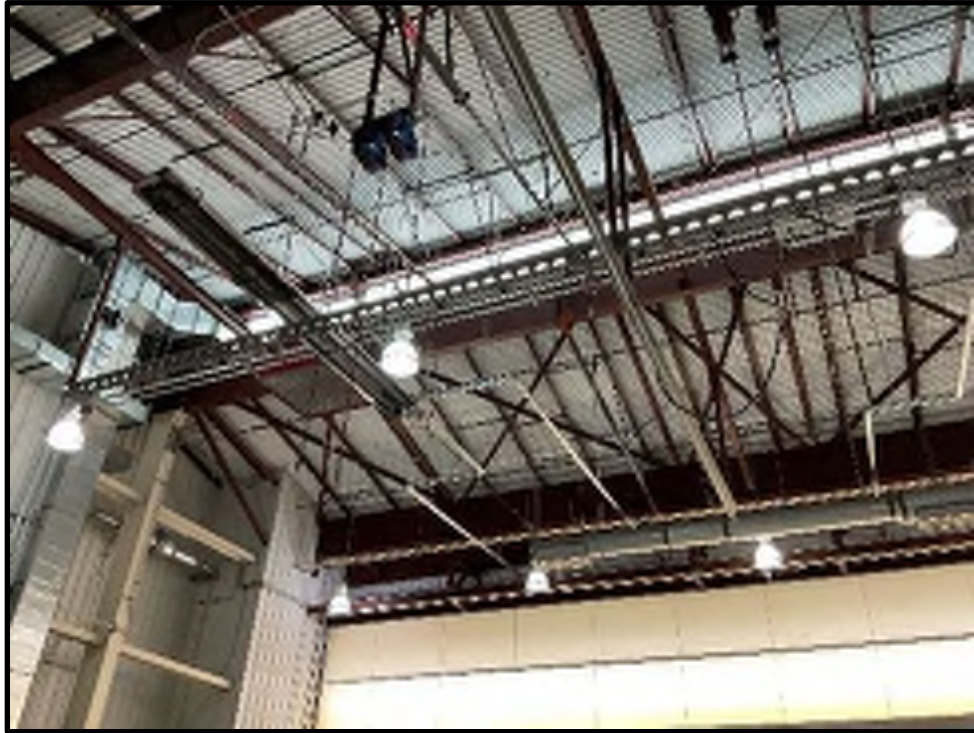
31 - B202 Existing Hangar Bay Ceiling
