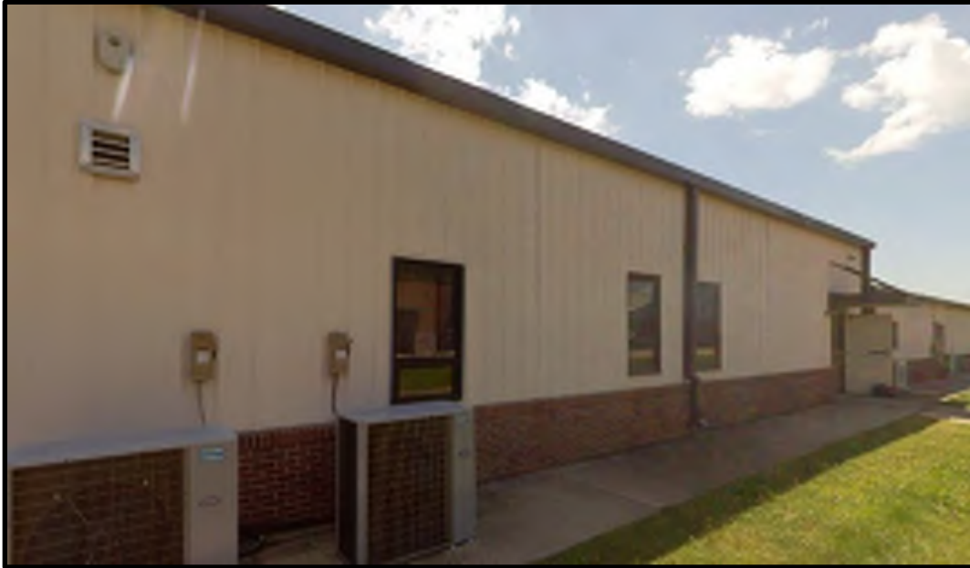
94 - B218 Exterior View #3
