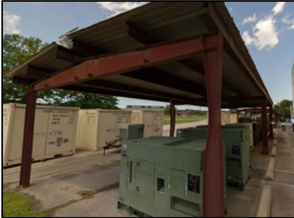
57 - B214 Exterior View #3
