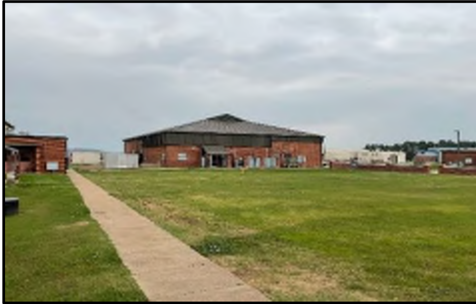
1 - B201 Exterior from Northeast
