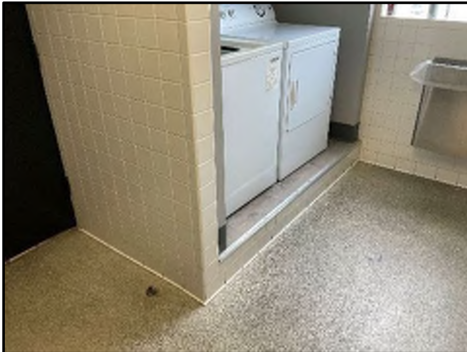
12 - B201 Washer and Dryer Curb
