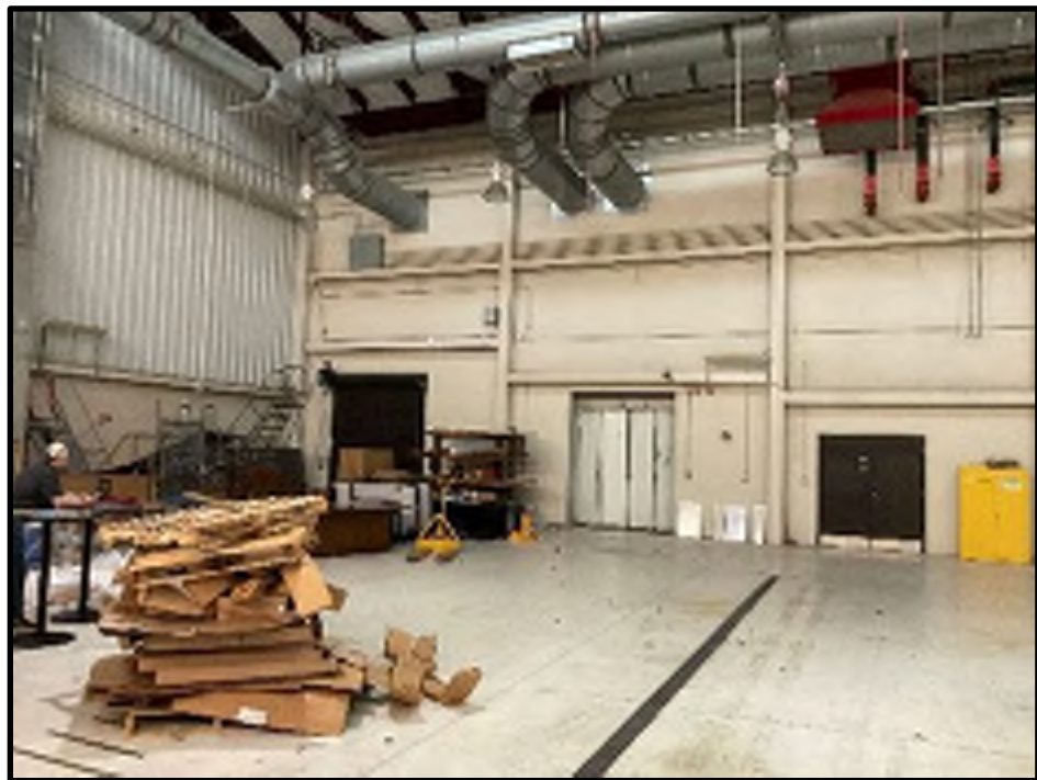
44 - B202 Hangar Bay 3 North Wall West Side
