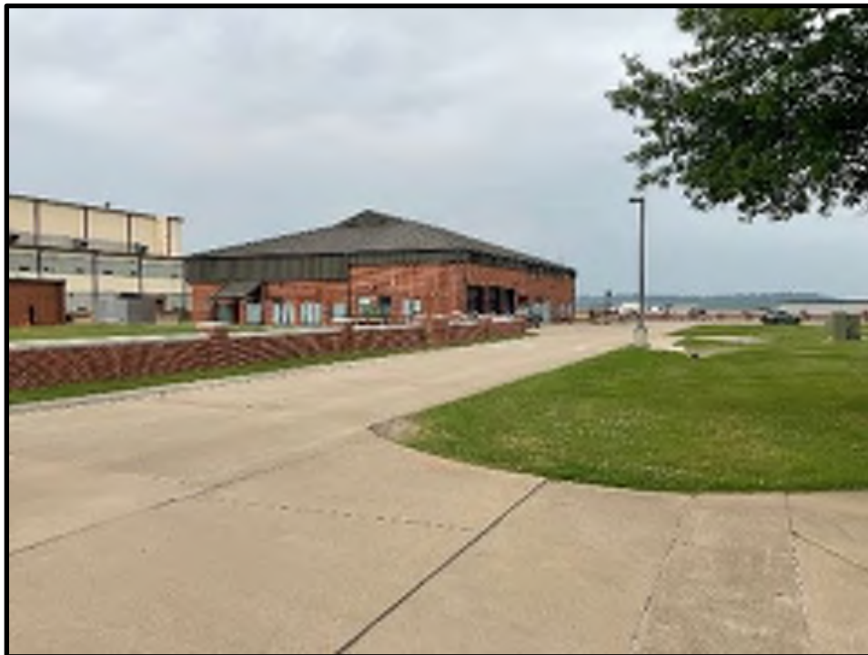
2 - B201 Exterior from Southeast
