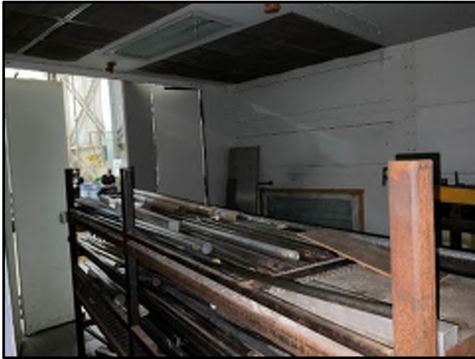
47 - B202 Paint Booth Interior
