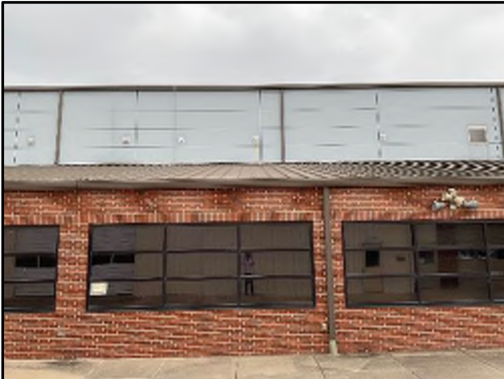
20 - B202 Existing Storefront Windows
