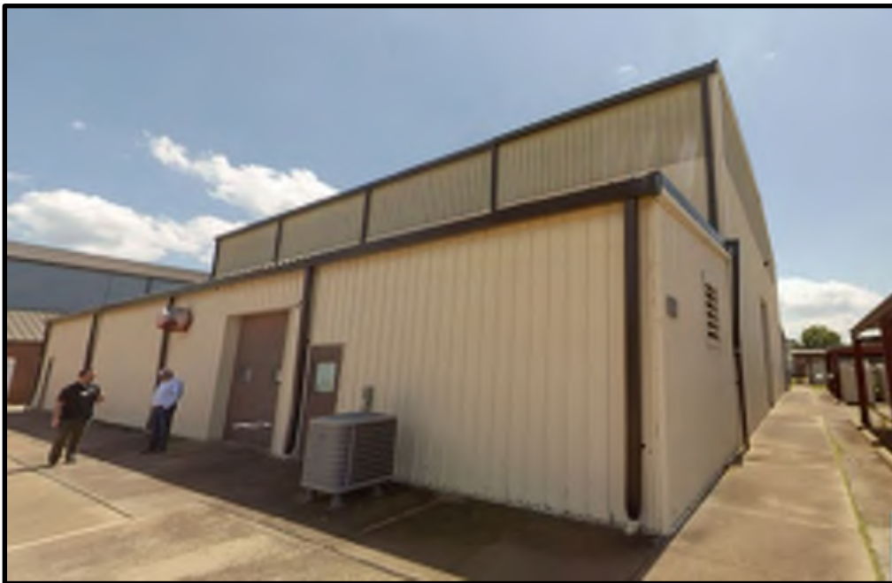
58 - B214 Exterior View #4
