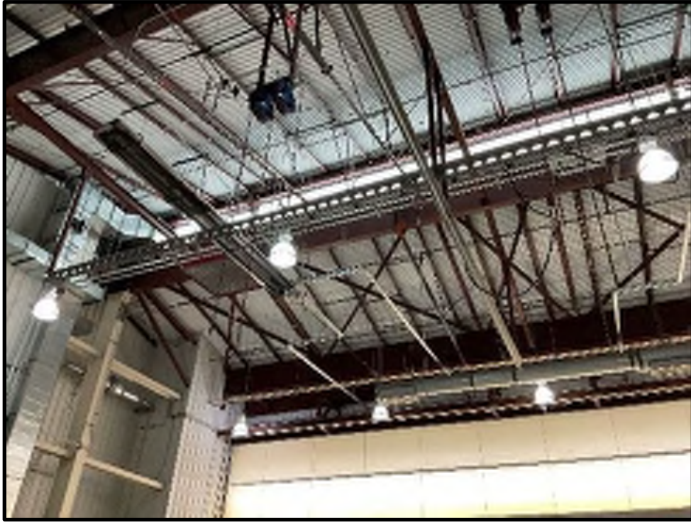
31 - B202 Existing Hangar Bay Ceiling
