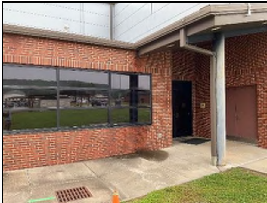
18 - B202 Covered Personnel Entry
