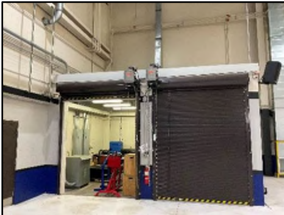
40 - B202 Hangar Bay 1 Storage Rooms
