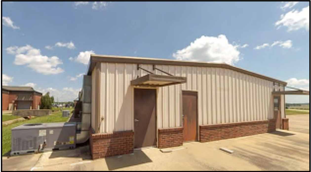
92 - B218 Exterior View #1
