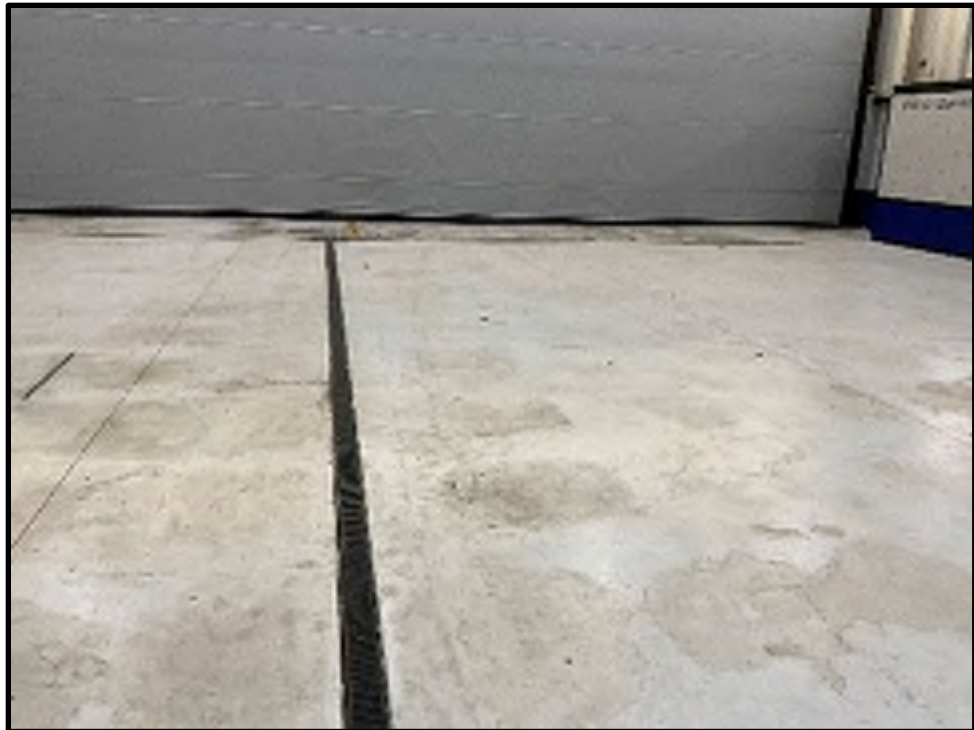
32 -B202 Existing Hangar Bay Epoxy Floor
