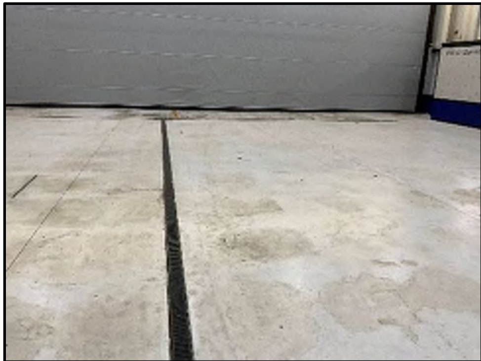
32 -B202 Existing Hangar Bay Epoxy Floor
