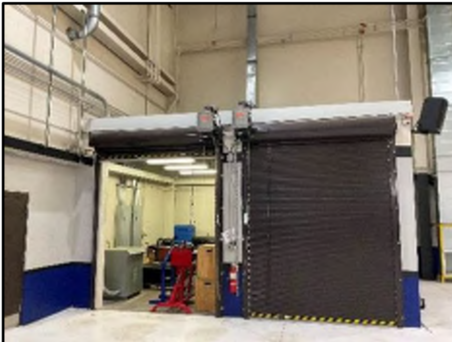
40 - B202 Hangar Bay 1 Storage Rooms
