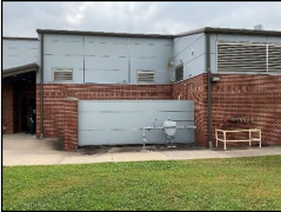
51 - B202 Utility Enclosure
