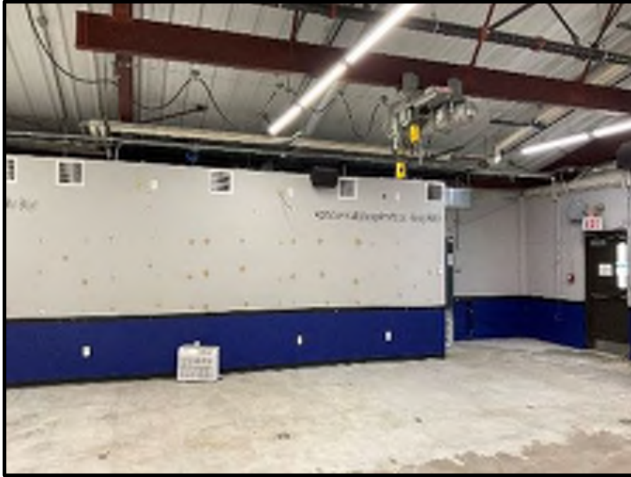
49 - B202 Tank Bay Screen Wall to be Removed
