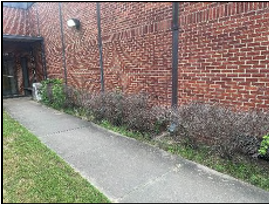
78 - B216 Downspouts by Addition
