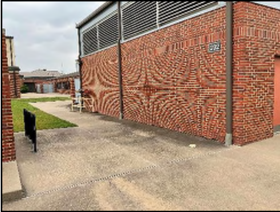
25 - B202 Northwest Corner
