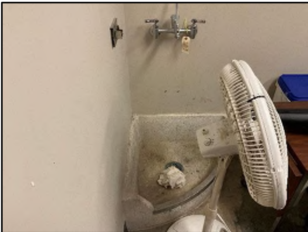
34 - B202 Existing Service Sink
