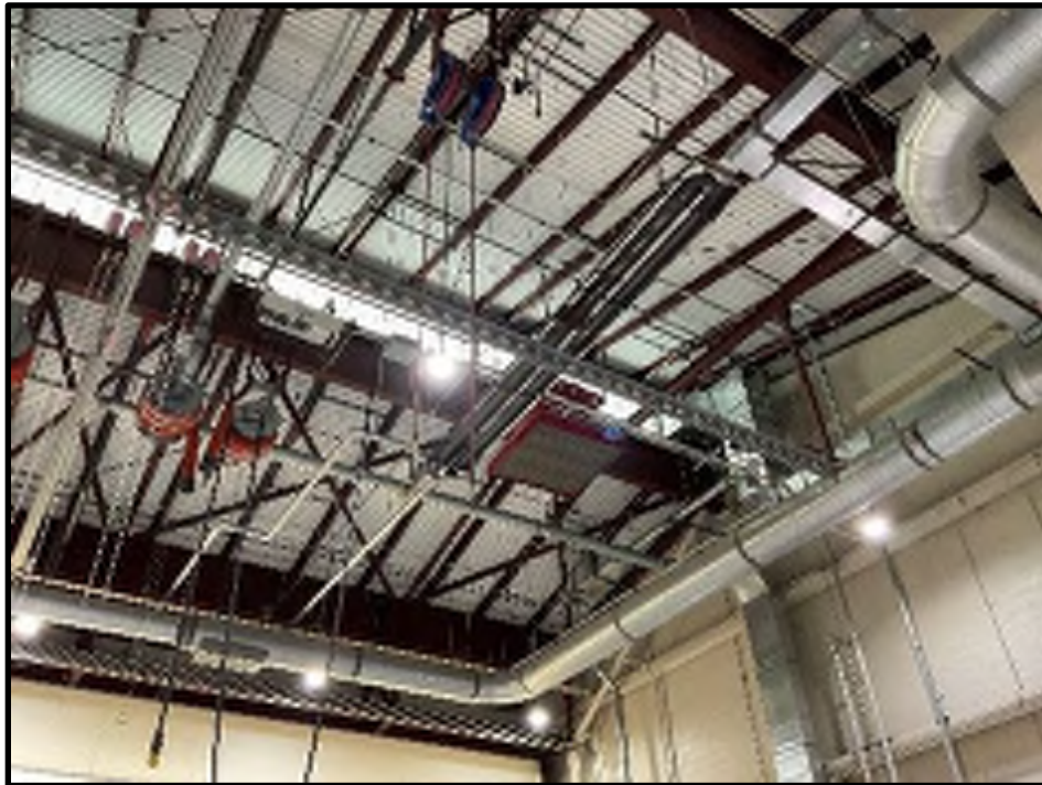
28 - B202 Bay 1 Ceiling
