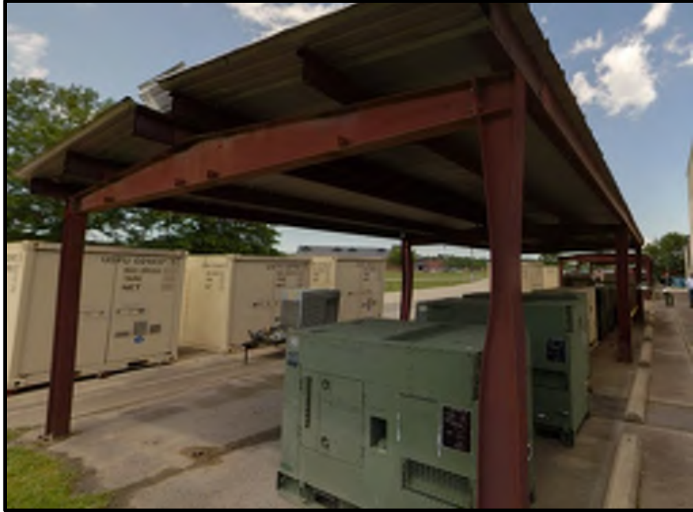
57 - B214 Exterior View #3
