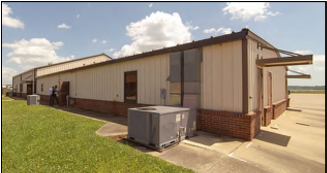
93 - B218 Exterior View #2
