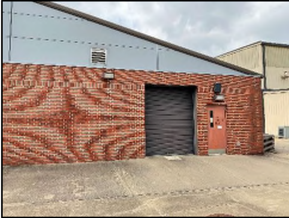
23 - B202 Exterior Tank Bay Doors
