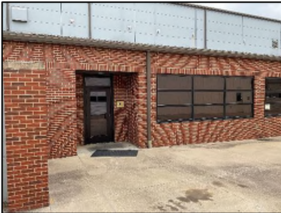
22 - B202 East Entry on North Side of Building
