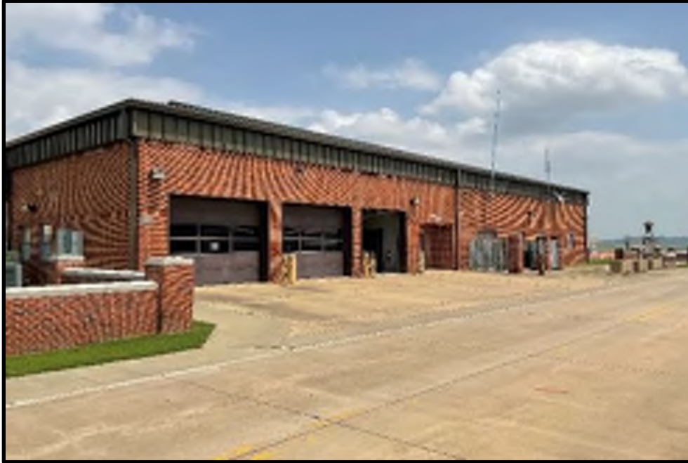
3 - B201 South Facade
