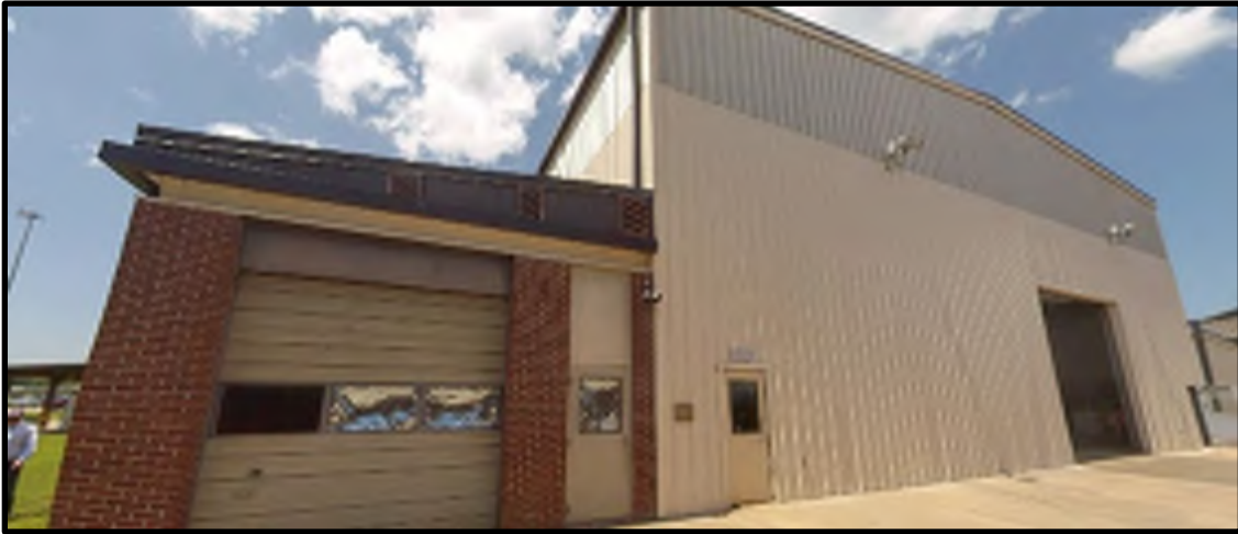
55 - B214 Exterior View #1
