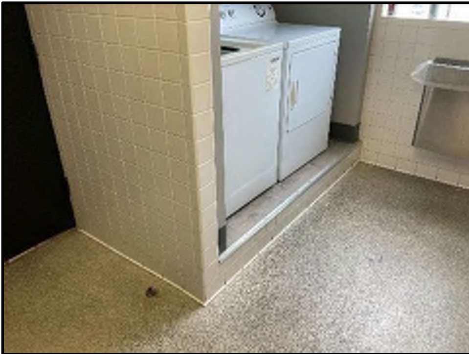
12 - B201 Washer and Dryer Curb
