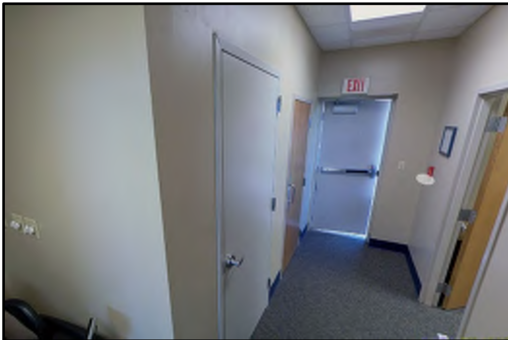
97 - B218 Comm Equipment at Entry
