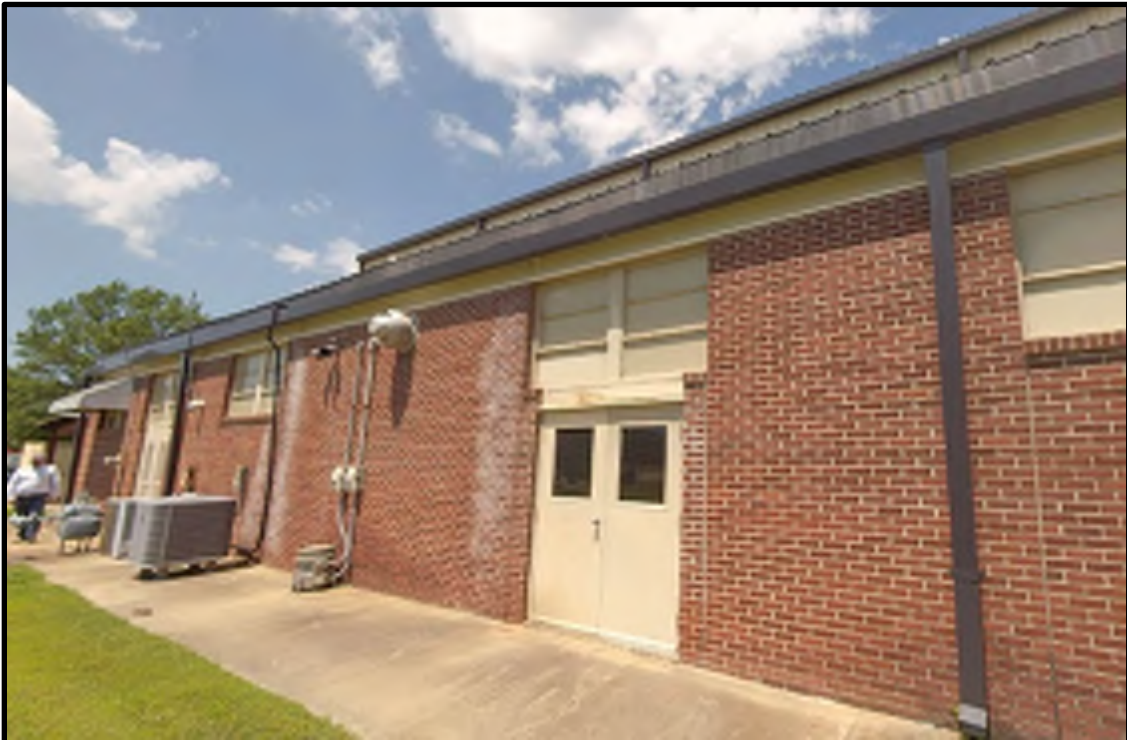
56 - B214 Exterior View #2
