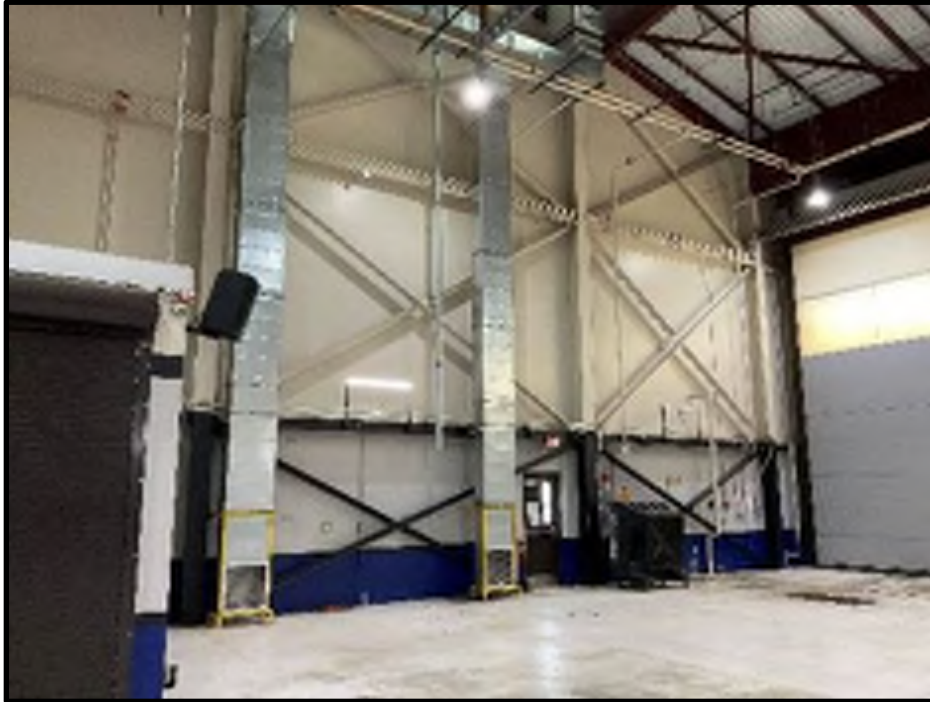
39 - B202 Hangar Bay 1 East Wall (Door to be Removed)
