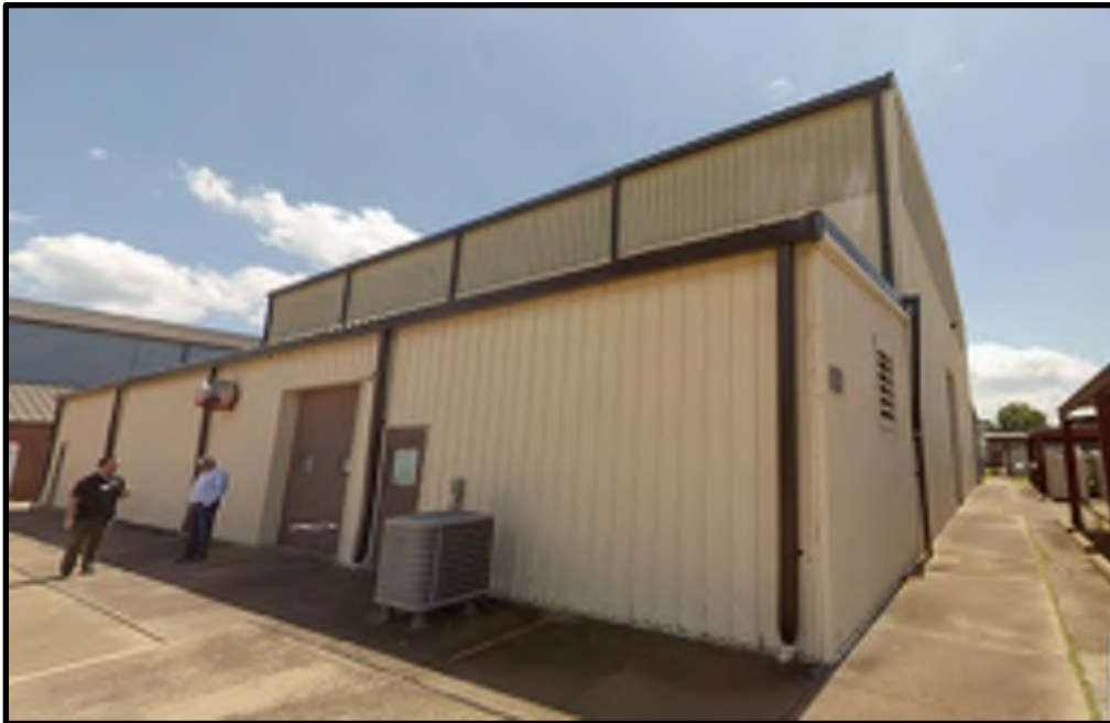
58 - B214 Exterior View #4
