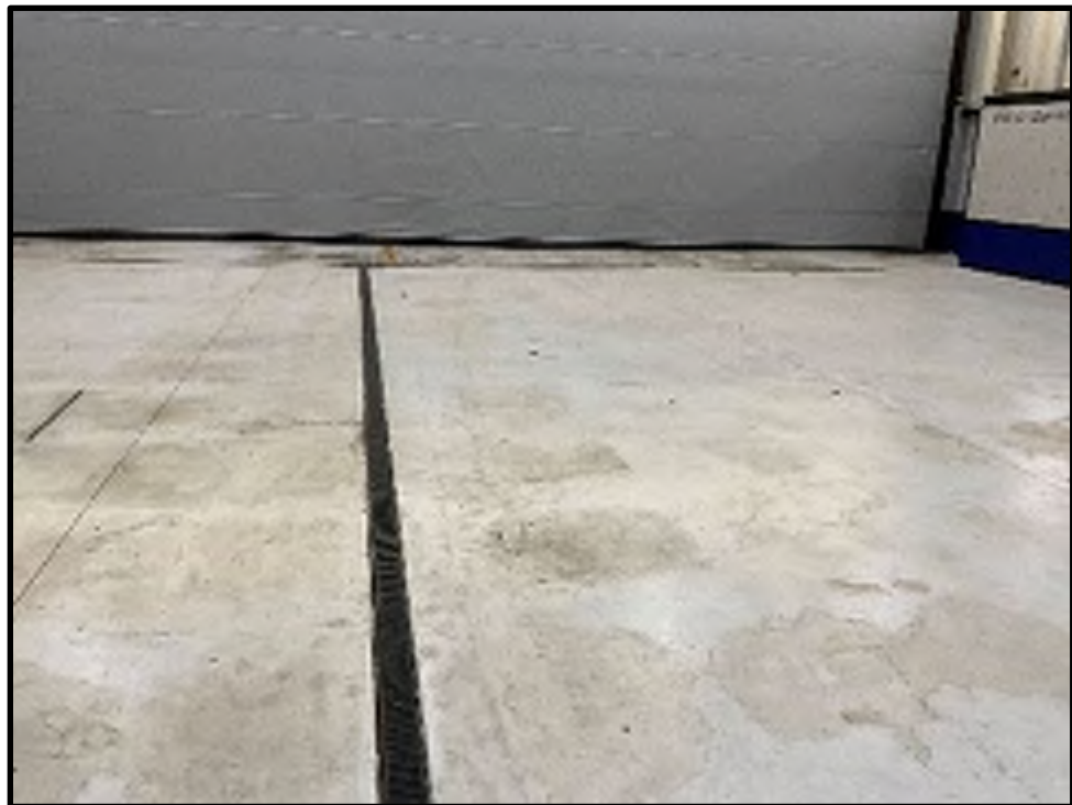
32 -B202 Existing Hangar Bay Epoxy Floor
