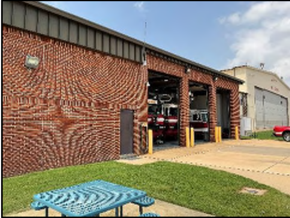
5 - B202 East Overhead Door Openings
