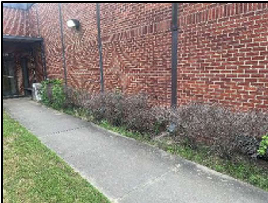
78 - B216 Downspouts by Addition
