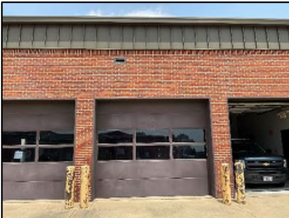
6 - B201 Infill South Doors
