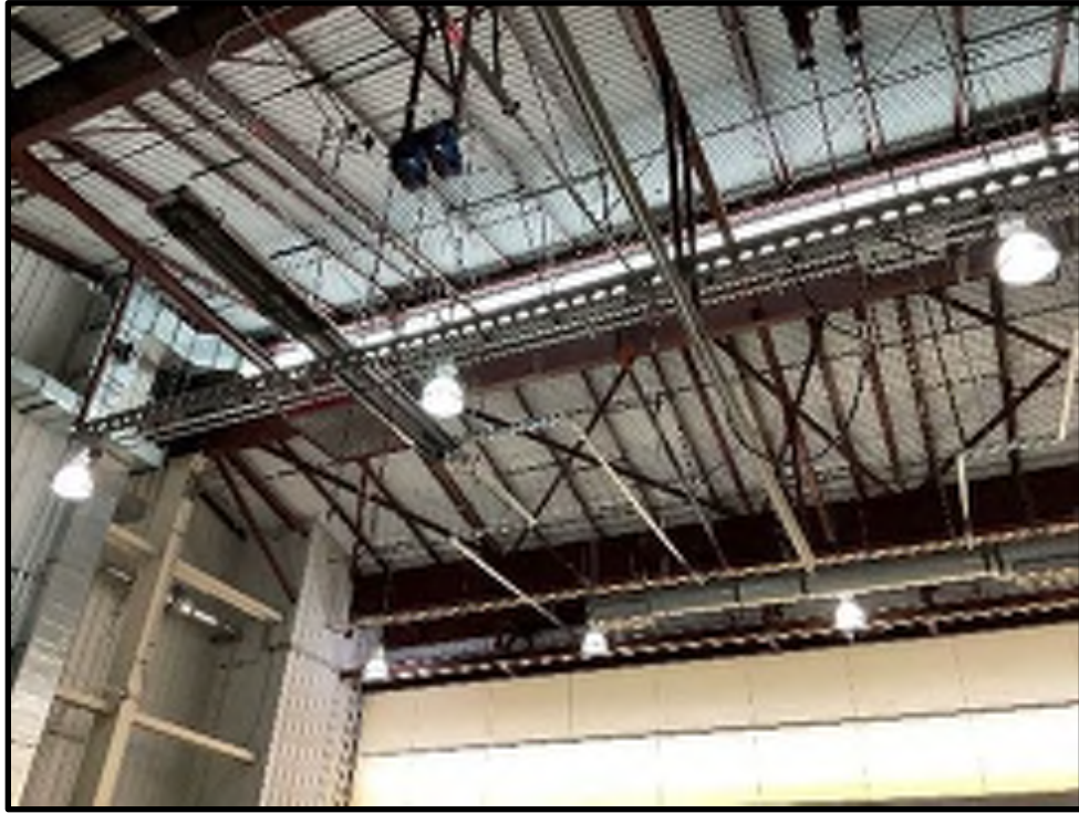
31 - B202 Existing Hangar Bay Ceiling
