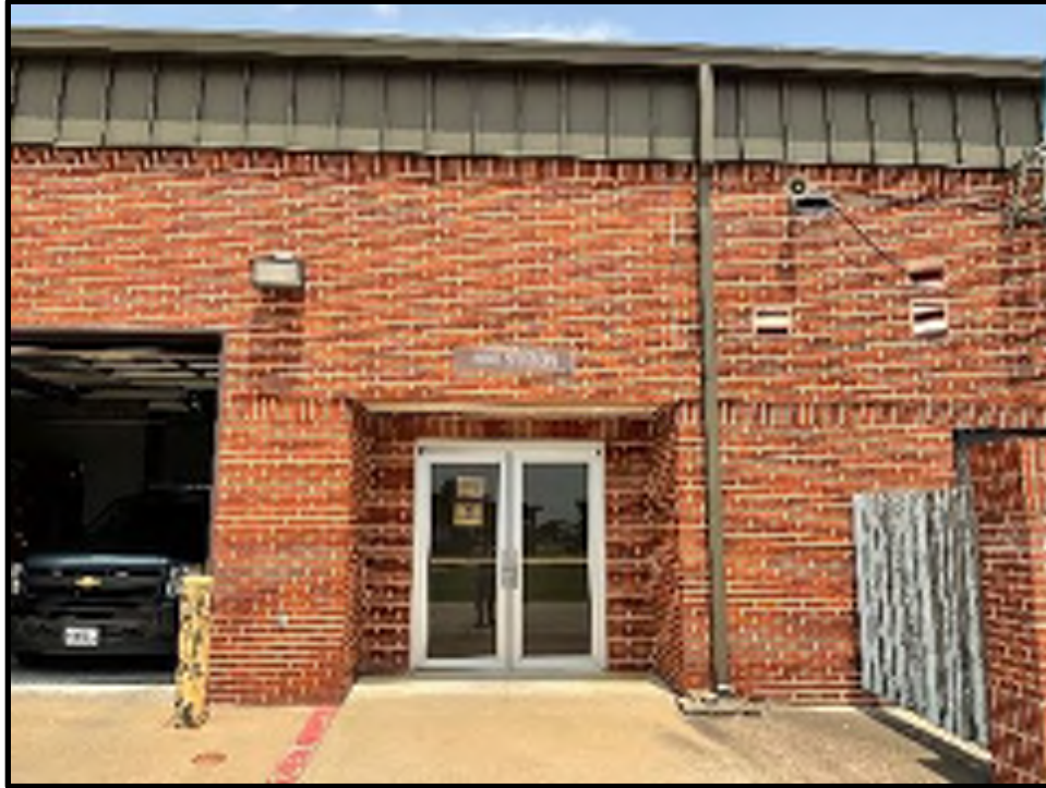
11 - B201 Infill South Doors
