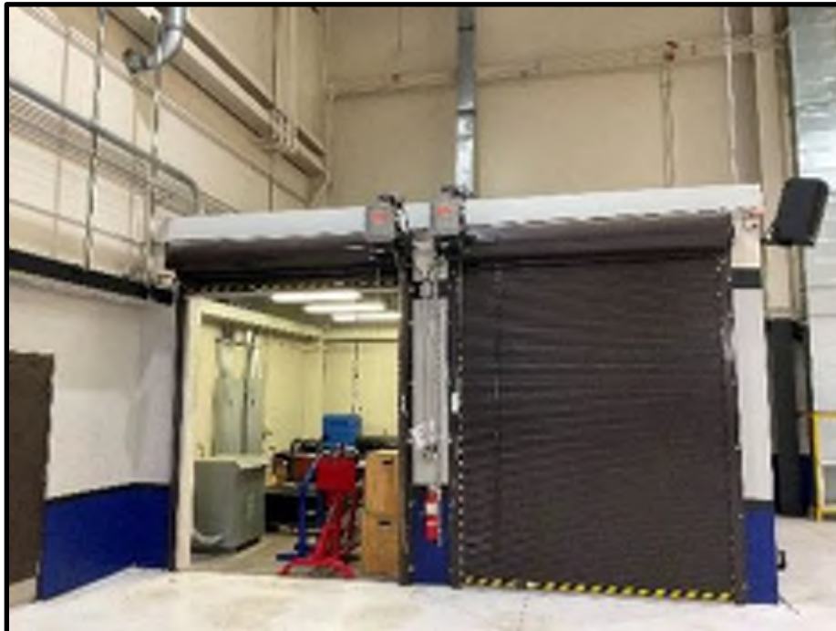
40 - B202 Hangar Bay 1 Storage Rooms
