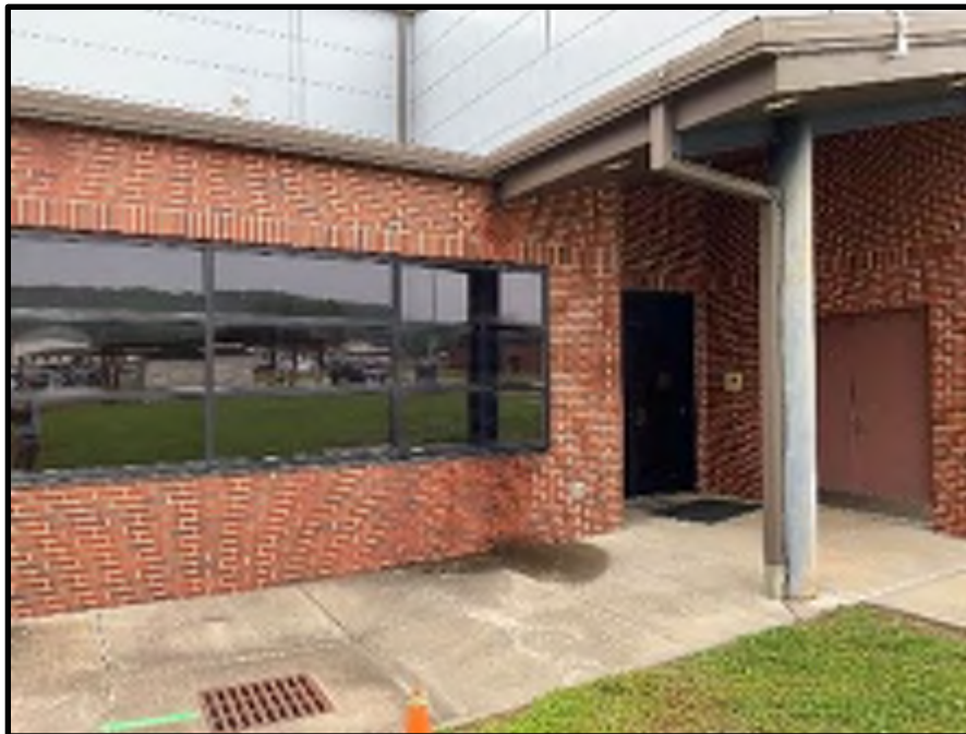
18 - B202 Covered Personnel Entry
