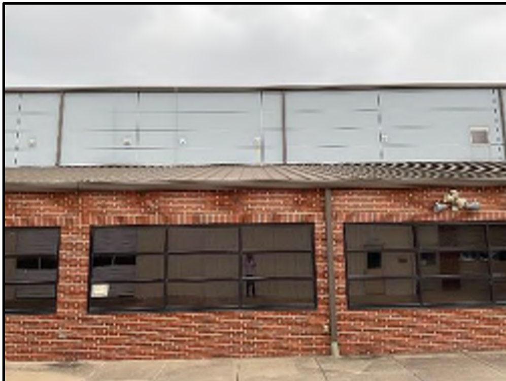
20 - B202 Existing Storefront Windows
