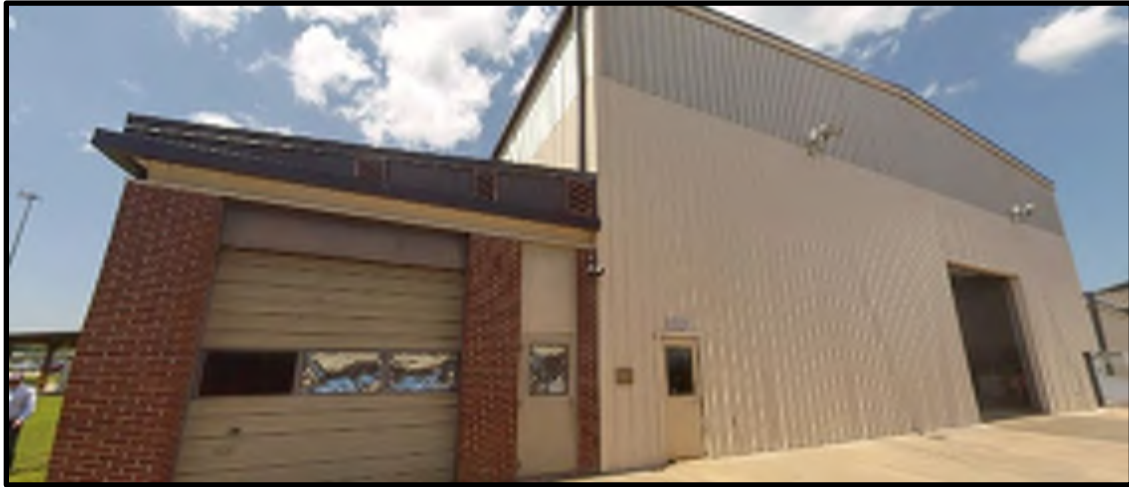
55 - B214 Exterior View #1
