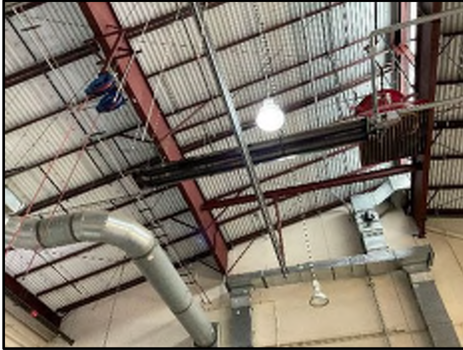
41 - B202 Hangar Bay 2 Ceiling
