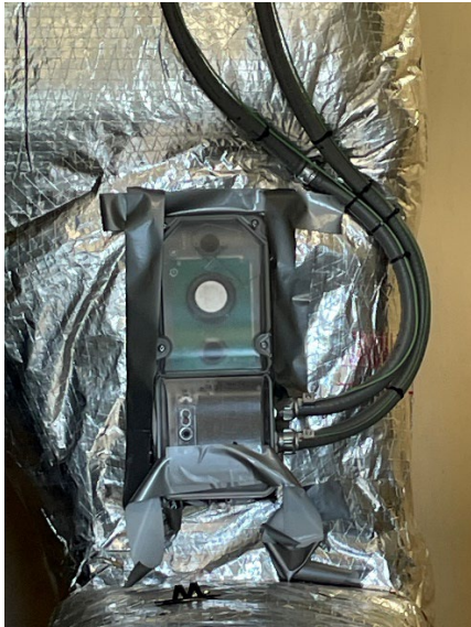
Figure 20: Duct Detector (Typical)
