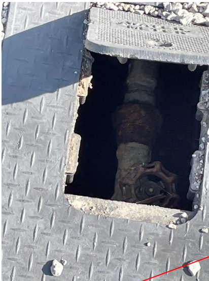
Figure 21: 2" Water line. Reroute Around Future Pad.
