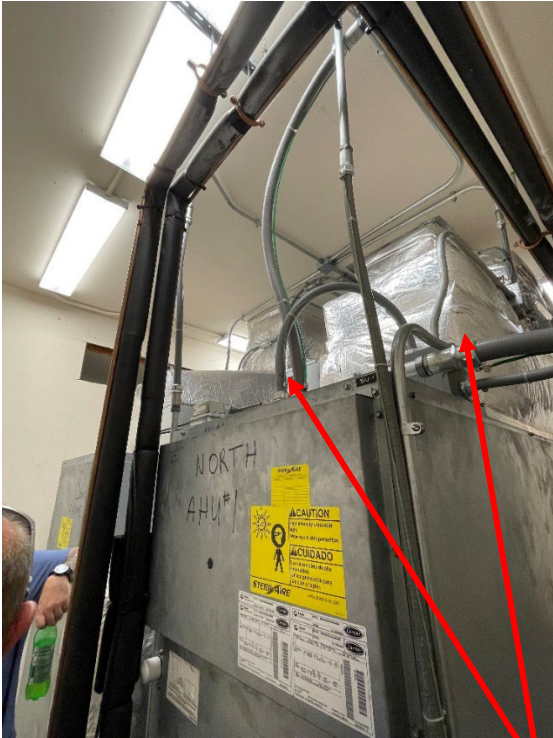
Figure 13: Typical Pics of Air handler units, Refrigerant Lines to be removed. Supply air ducts visible going above ceiling.
