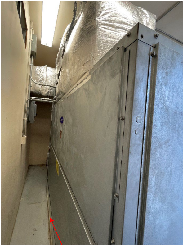
Figure 12: Typical Pics of Air Handler Units (To Be Removed) Remove concrete pad.
