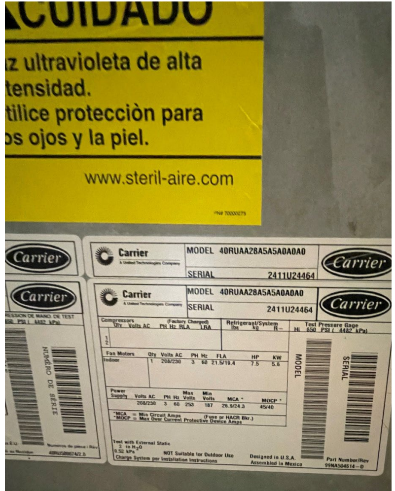
Figure 4: AHU#1 Nameplate
