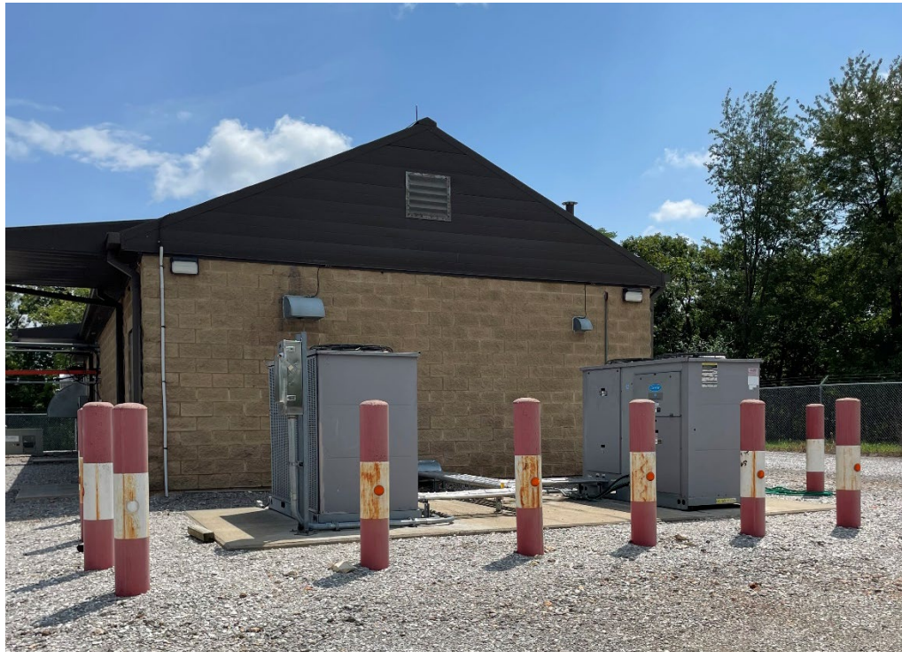
Figure 3: Outside Facility View
