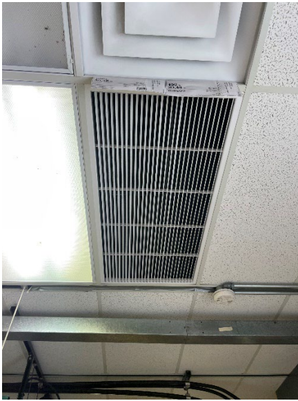
Figure 25: Blank Cover Duct Openings
