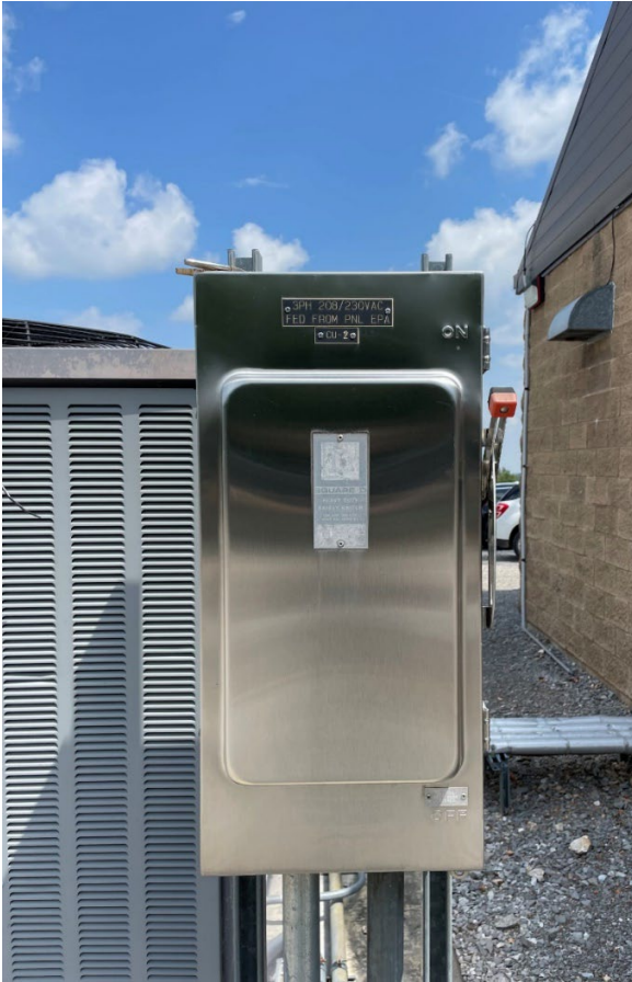
Figure 5: Existing NEMA 4X Disconnect Switch
