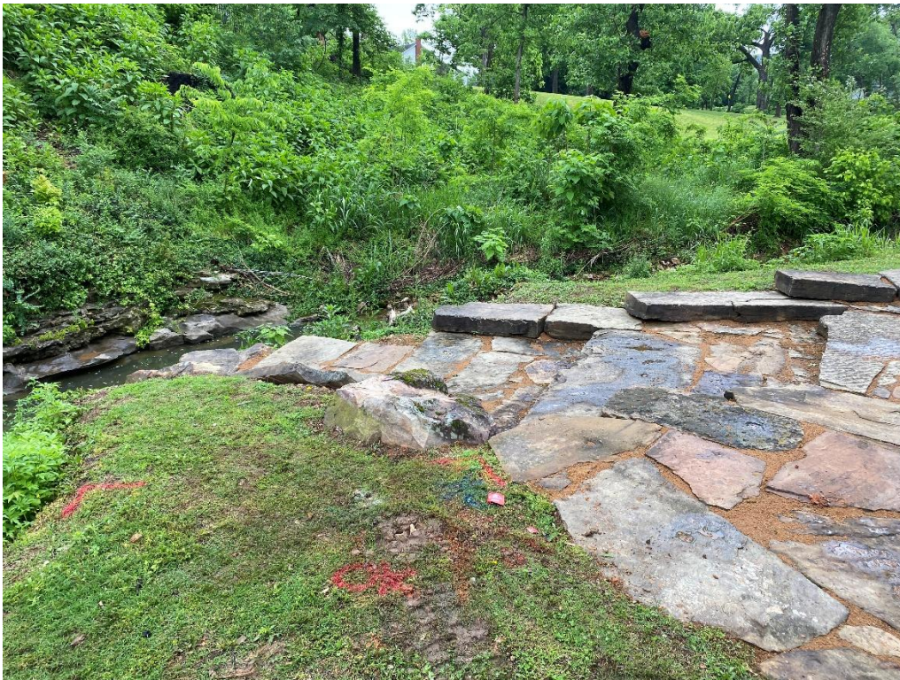
Figure 1: Northwest side boundary of the site looking east (facing the proposed location of the pedestrian bridge)
