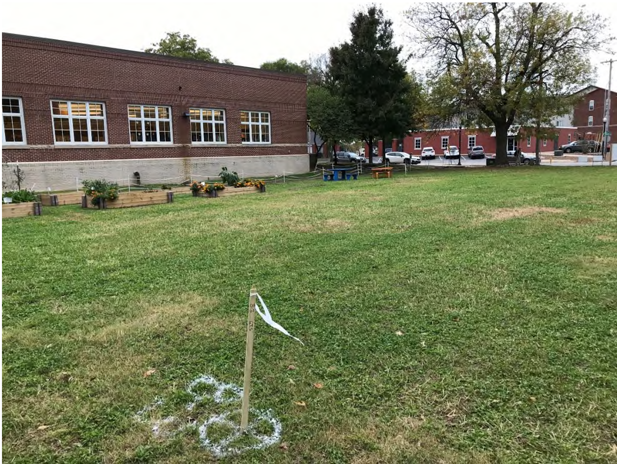
Photograph 1 – Looking Southwest with Boring B-3 in foreground and existing library in background, left
