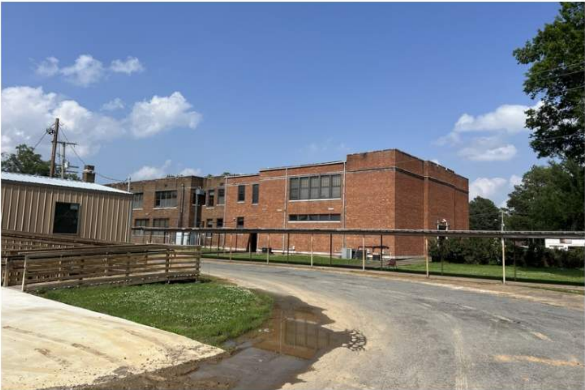
Photograph 2: West Side of Existing Building
