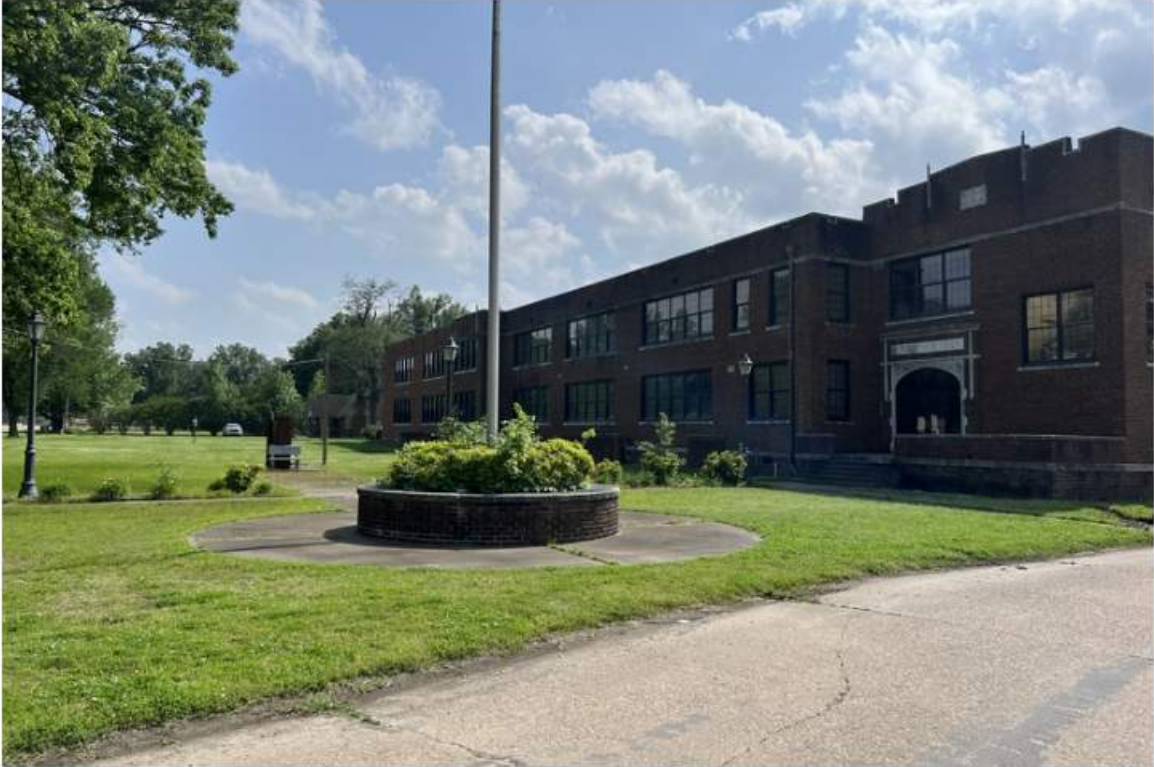
Photograph 1: East Side of Existing Building
